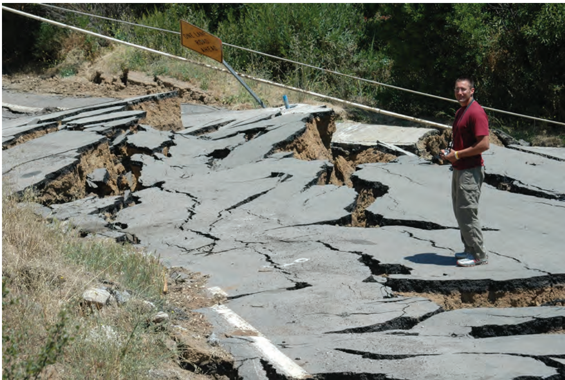
Figure 1.2 Society needs the input of geoscientists. A landslide destroyed this important access road in southern California that cost many millions of dollars to repair. Geoscientists provide society with the expertise needed to effectively address challenges related to energy, supply of industrial minerals, fresh water, climate change, and natural hazards ranging from landslides and floods to earthquakes and volcanic eruptions.
